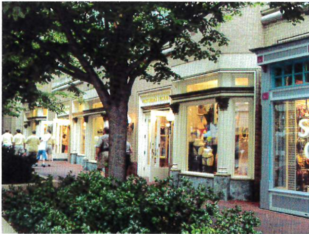
The front elevations of these buildings show a mixture of structure articulation, appropriate window proportion, and quality building materials.
