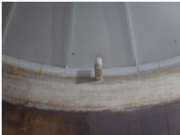
45) The overflow elbow is in good condition.
