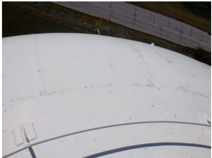
14) The roof coating has faded but there is no significant deterioration.
