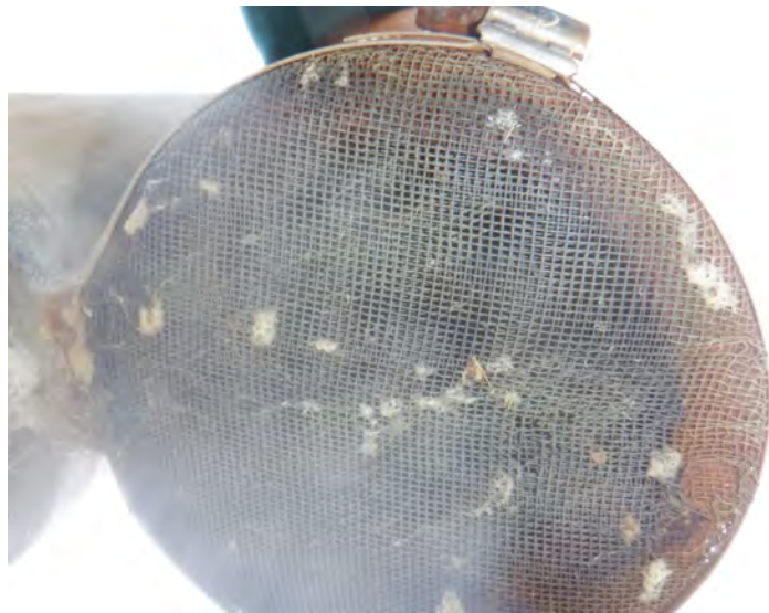
5) The roof vent screen is intact.
