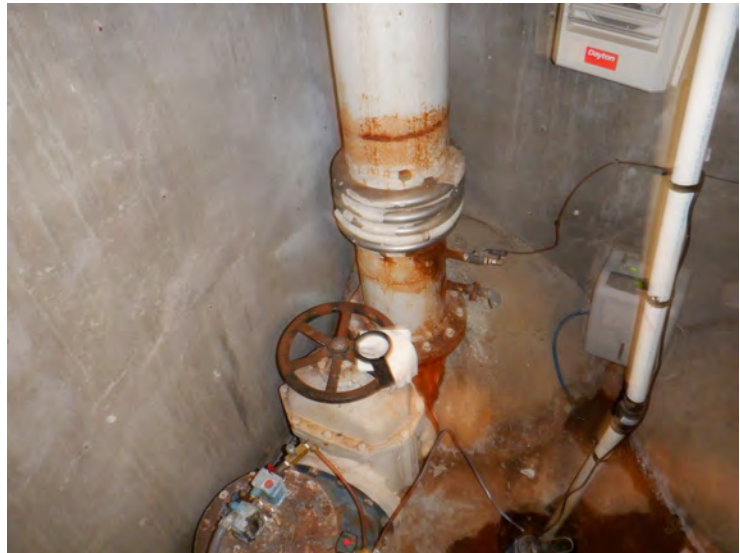
68) The bellow type expansion joint is in good condition.
