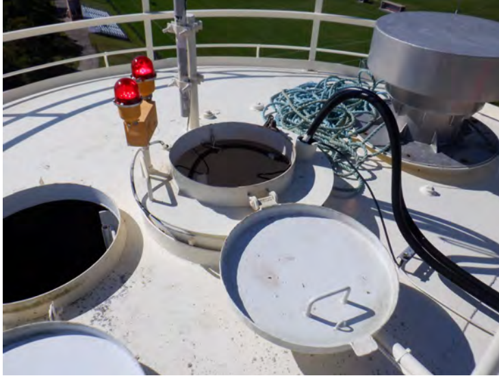
19) The dry interior roof hatch is in good condition.
