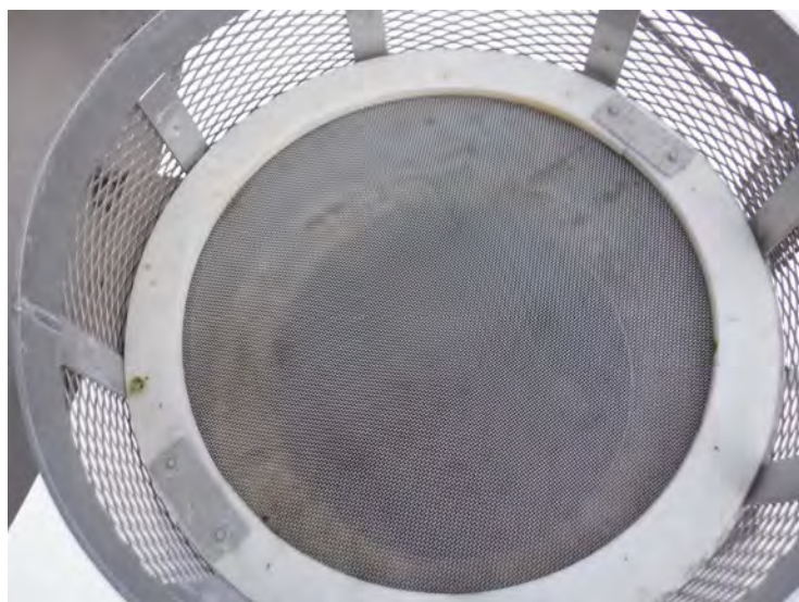
36) The interior screen is in good condition.
