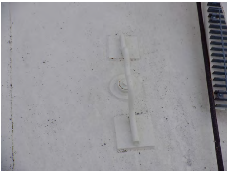
30) Some of the roof rigging couplings have safety clips that are in good condition.
