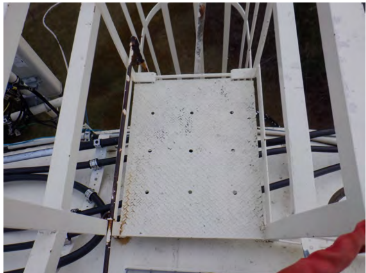
23) The step-off platform is in good condition.
