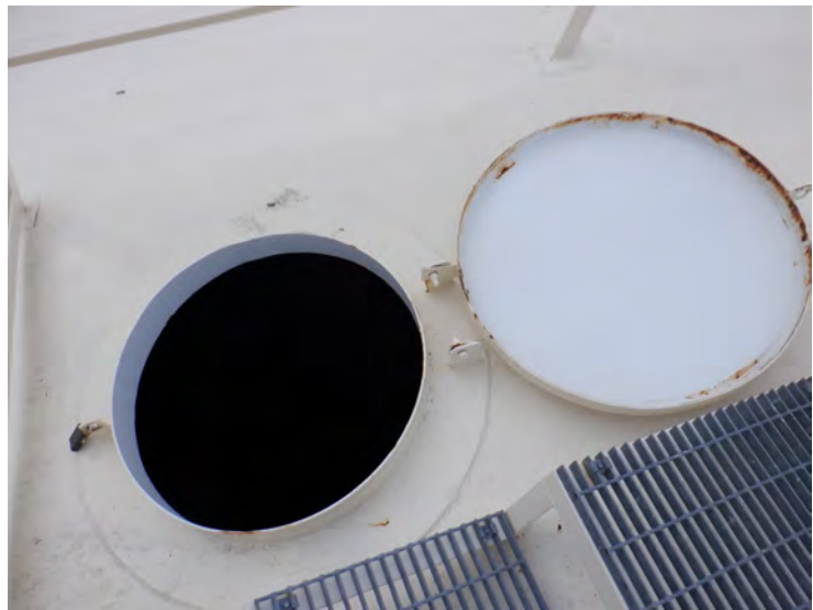
38) The roof hatch is in good condition.
