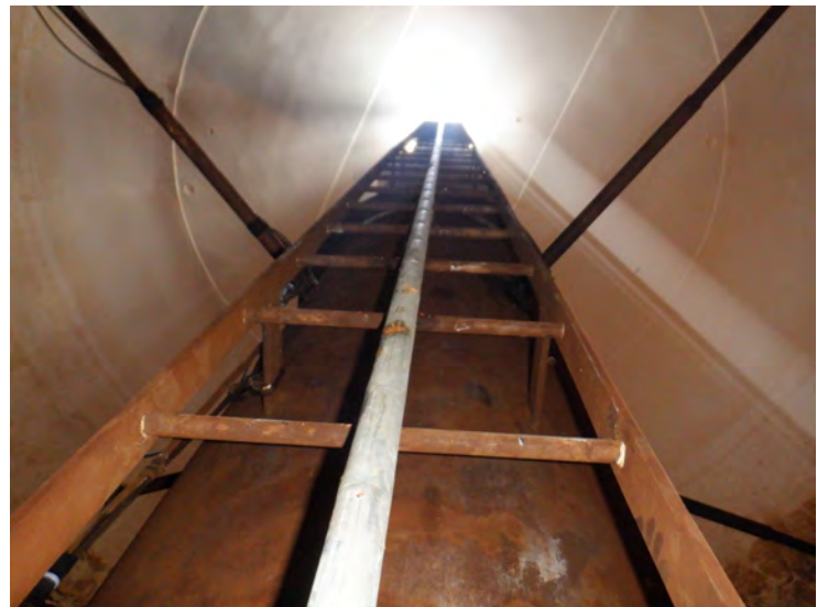
59) The wet interior ladder is in good condition. The ladder is equipped with a fall prevention device.
