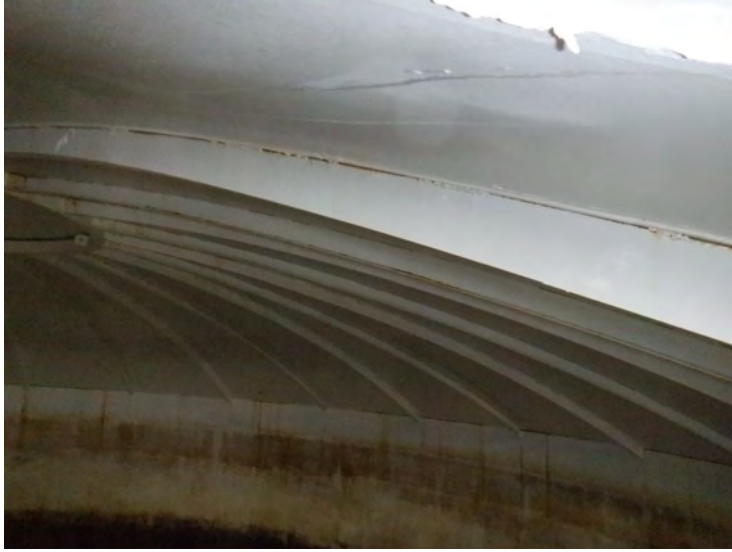
43) The roof stiffeners are in good condition.
