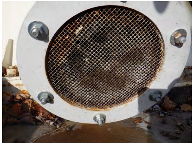
5) The screen at the overflow pipe discharge is intact with no gaps.
