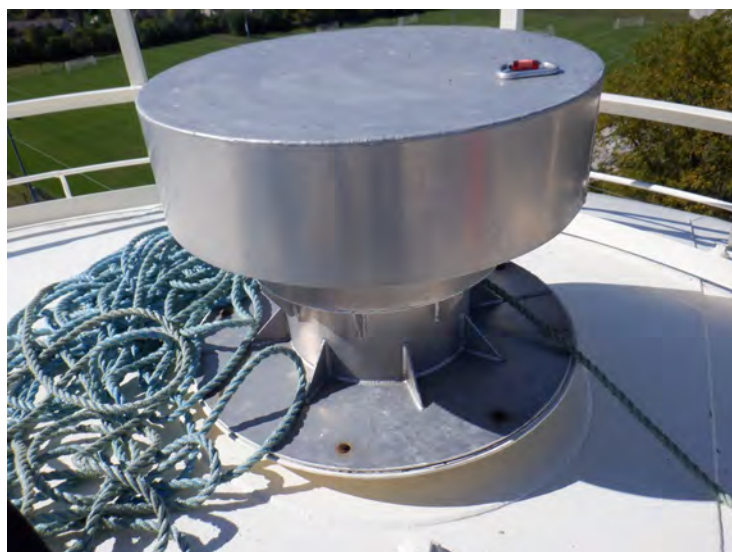
21) The roof vent is in good condition.
