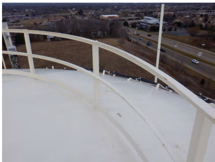
27) The center handrail is in good condition.
