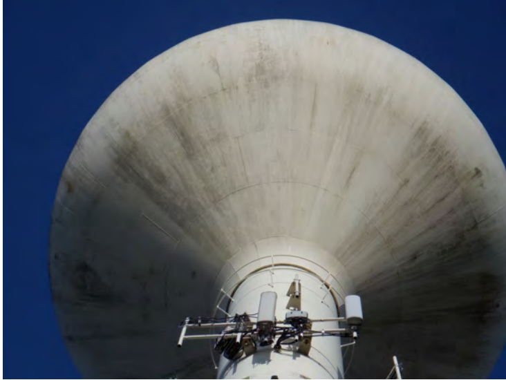
16) The bowl is covered with moderate mildew growth.
