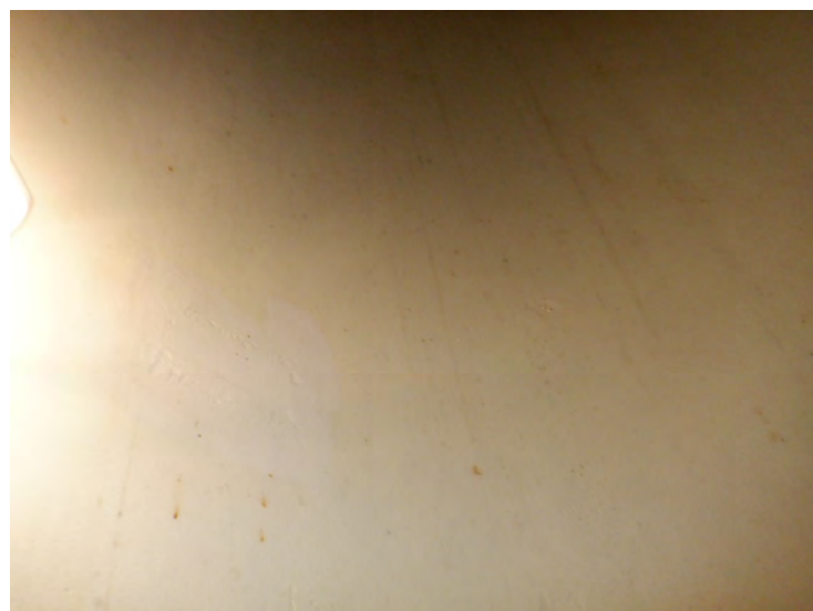
39) The dry riser coating is in good condition overall.
