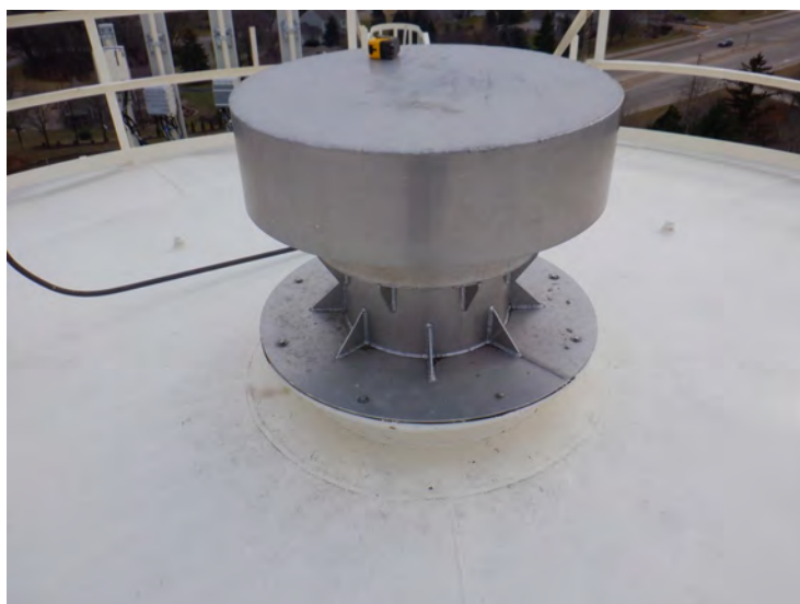
33) The roof vent is in good condition.
