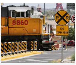
Two 100 ft. sections of QWICK KURB Continuous Curb, can be installed in about three hours at a fraction of the cost of other SSMs, with little maintenance thereafter. Additional road work or crossing closures are not required to install the system.
