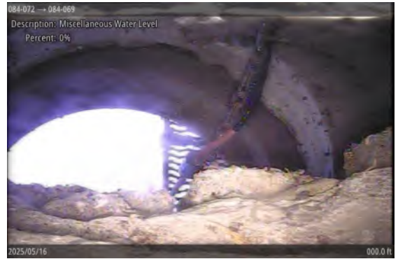
Miscellaneous Water Level at 000.0 ft
