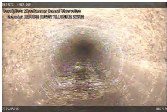
Miscellaneous General Observation at 007.5 ft | REDOING SURVEY TILL UNDER WATER
