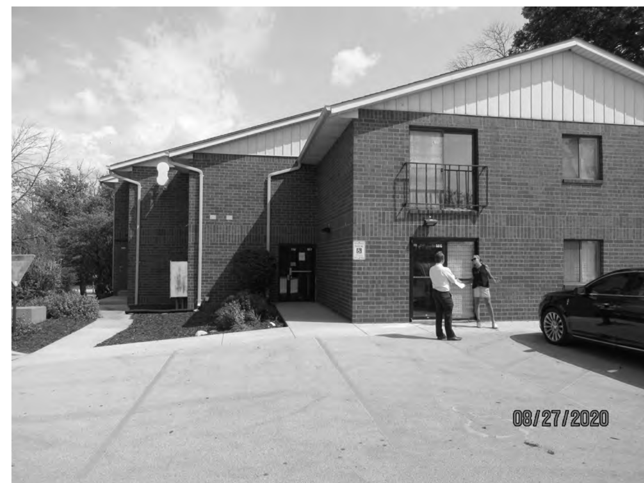
EXISTING MAIN ENTRANCE
