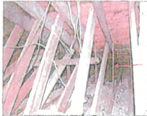
32. View into attic perimeter. Note vertical plaster supports
