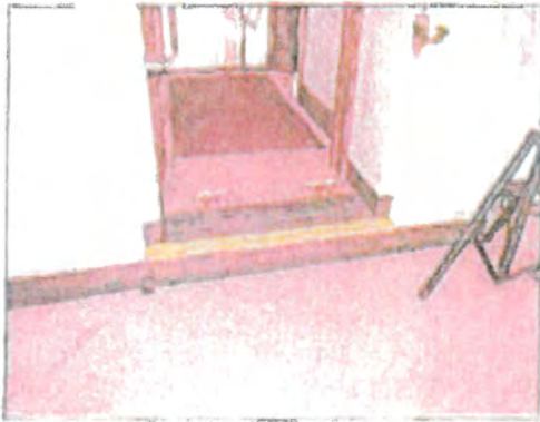
15. Change in floor elevation from church into annex
