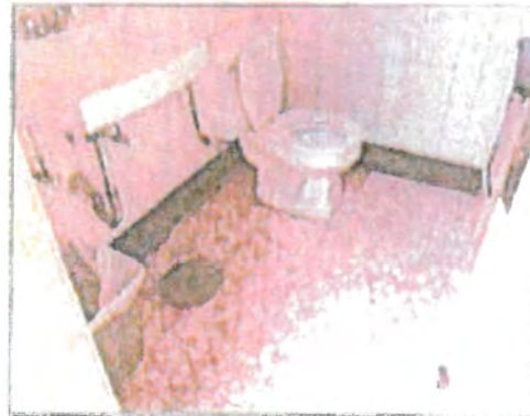
34. Existing ladies' room.
