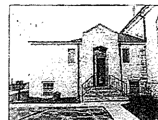
14. Annex entrance, south elevation. Note the tip hazard painted yellow.
