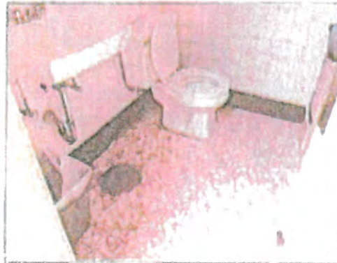
22. Existing ladies room.
